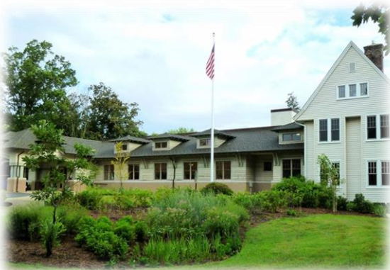
Rain garden at Monmouth County Library's Ocean Township branch
