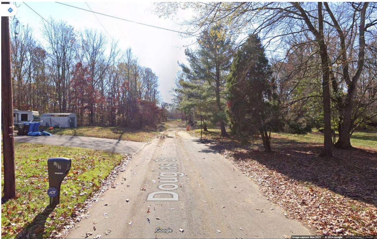
END OF IMPROVED SECTION OF DOUGLAS STREET (FACING SOUTH)
